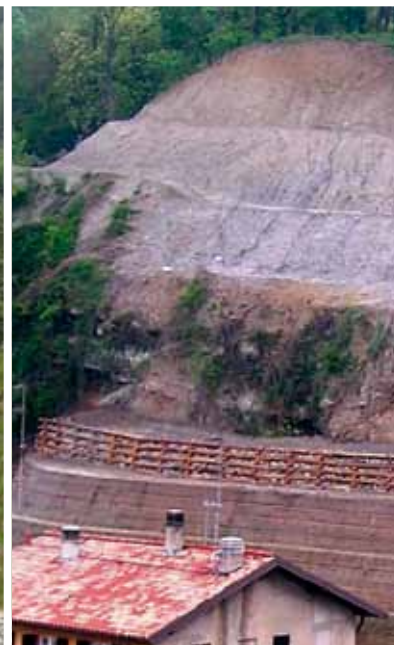
Construction and re-profiling of a 12.5m high slope close to a small residential area close to Lecco, Italy.
