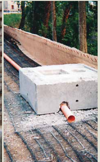
Before filling the last course of the embankment, it is possible to create recesses to take street lighting.
