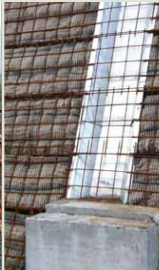
Placement of metallic tiles for drainage of surface waters.
