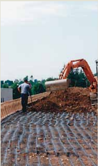
The geogrids are placed at the front or back depending on whether the section is convex or concave.
