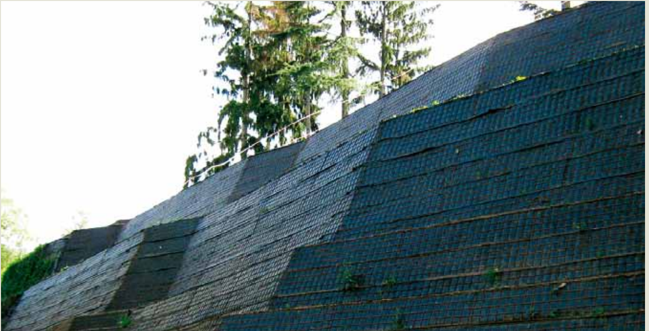
Tenax Rivel structure installed using a weed control fabric and awaiting ornamental planting.
