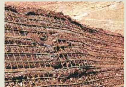
Minimum extrusion of the downhill face of the embankment
