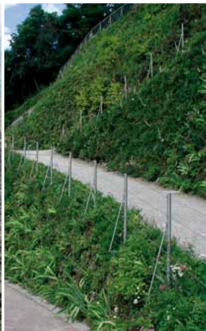
Terraced gardens using TENAX reinforced slopes at Merano Botanical Garden, Italy.
