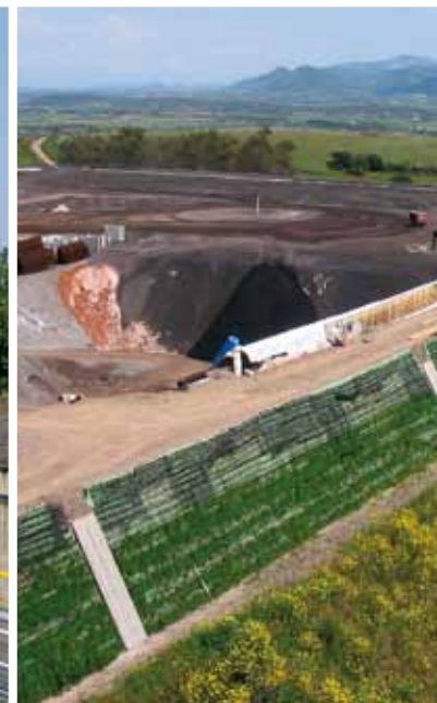
Construction of four soil reinforced trapezoidal perimeter dikes to retain waste within Genna Luas landfill, nr.Cagliari, Italy.
