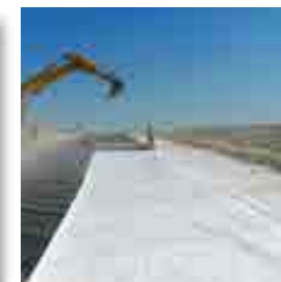
Installation of the Geocomposite for drainage of infiltrating rain water
