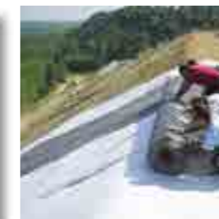
Installation of the Geosynthetic Clay Liner or Geomembrane
